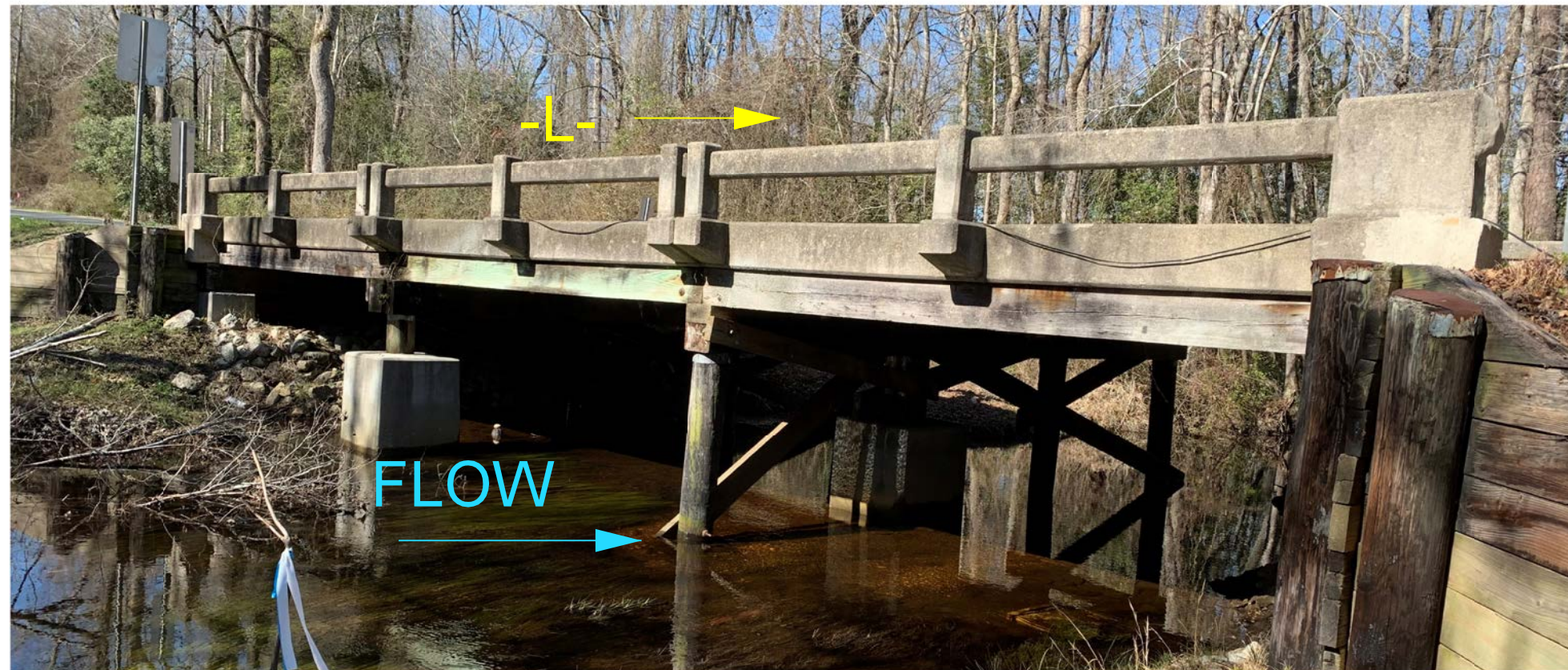
LOOKING DOWNSTREAM FROM RIGHT SIDE OF END BENT 2
