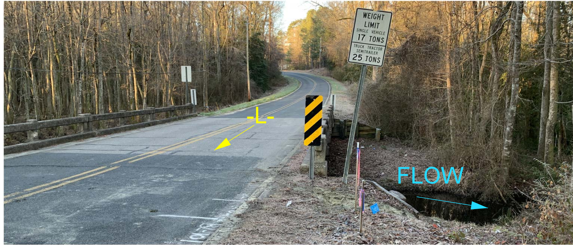
LOOKING WEST FROM END BENT 2 TOWARD END BENT 1
